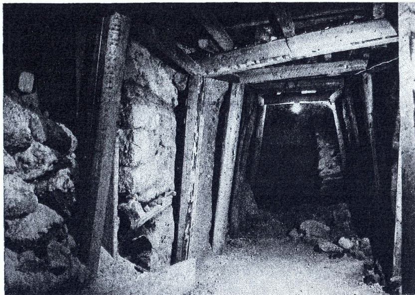
a. Excavation by tunnelling. Walls of buildings appear on each side (1969).
